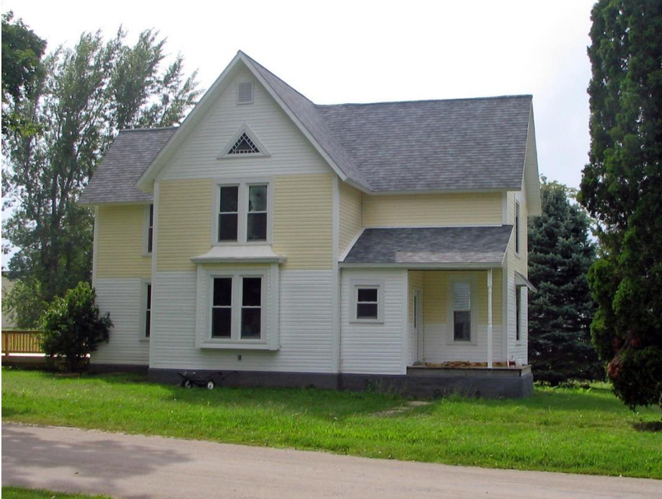
The Sim Town House in 2008 after renovation was completed.
