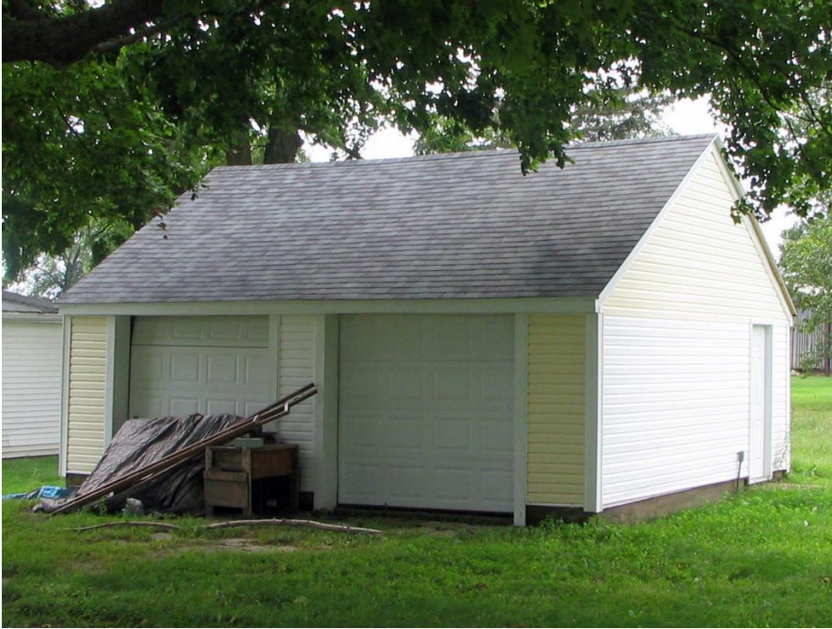
The garage that Duncan Wasson built was also repaired and updated.
